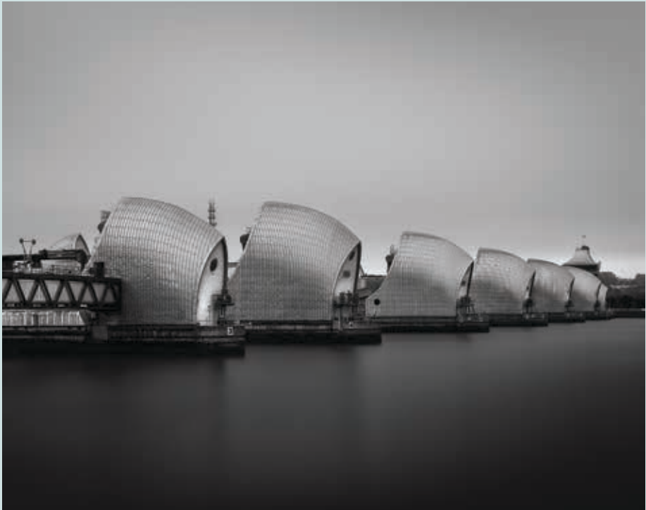
The Thames Flood barrier outside London City
